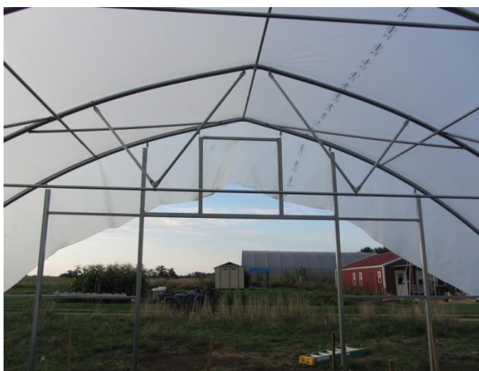
Metal End Wall Framing
