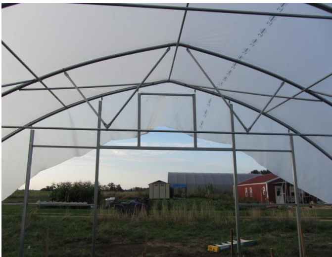
Metal End Wall Framing
